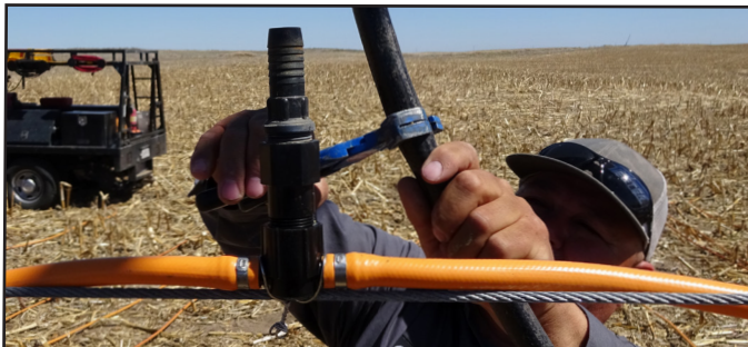
C) Cut to length 3/4" inch hose and connect to barb fitting on top of dual valves with 3/4 inch clamp
