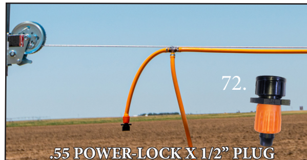
B) Install manifold hose into power-lock fittings and wire tie.
