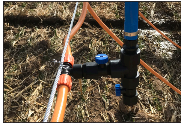
B) Install manifold hose into power-lock fittings and wire tie.
