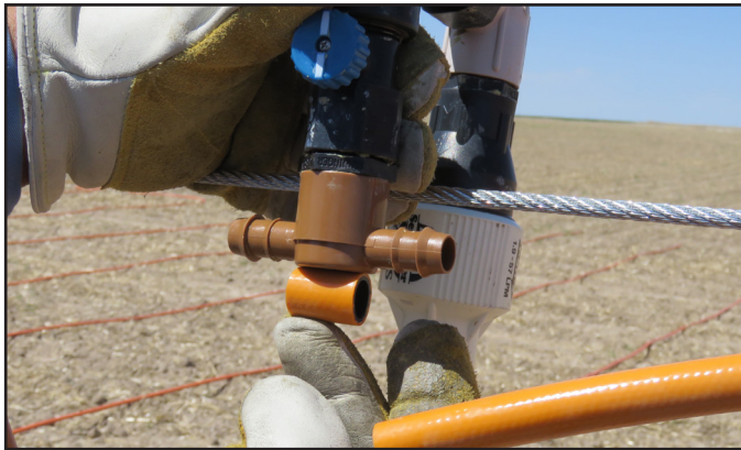
A) Find location of existing drop hose and cut 1-2" on manifold spacing. (Cut length varies depending on the Tee fitting).
